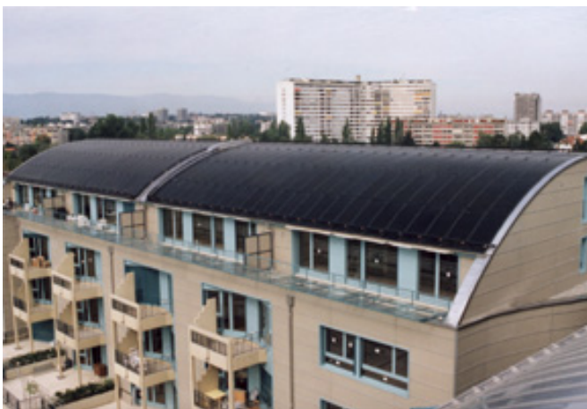
Figure 14: Selective, unglazed collectors (energie solaire, Toiture Solaire AS). The collectors are part of the building and can be used for SDHW /Ene05/ especially in areas with limited wind.
