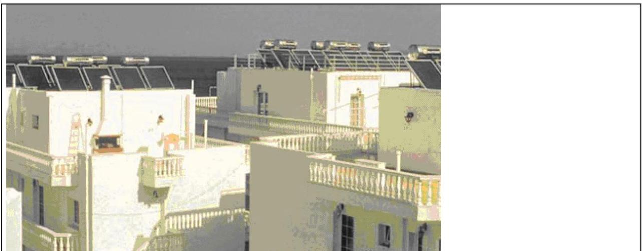
Figure 1: Reference system: thermosyphon solar water heaters
