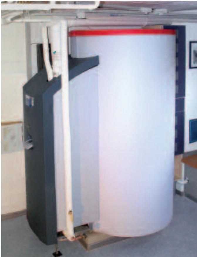
Solar combisystem as a pre-fabricated unit reduces the number of connections to be made on site SOLVIS
